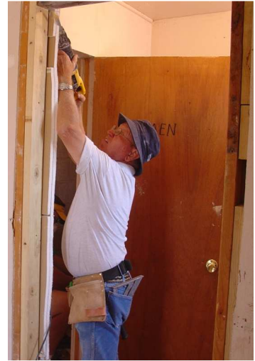
Rick takes care of the bathroom remodeling project
