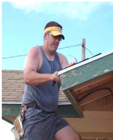
Andy takes care of the missing shingles
